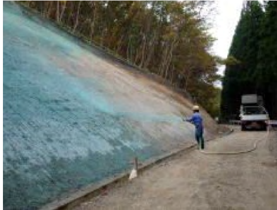
PHOTO 10.2-2 WORKING EXAMPLE OF SOWING
