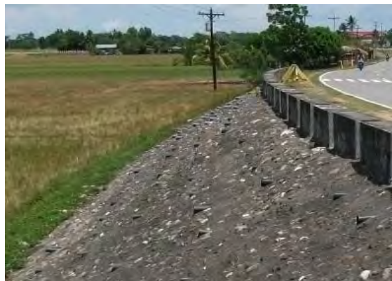
PHOTO 10.2-9 WORKING EXAMPLE OF GROUTED RIPRAP
