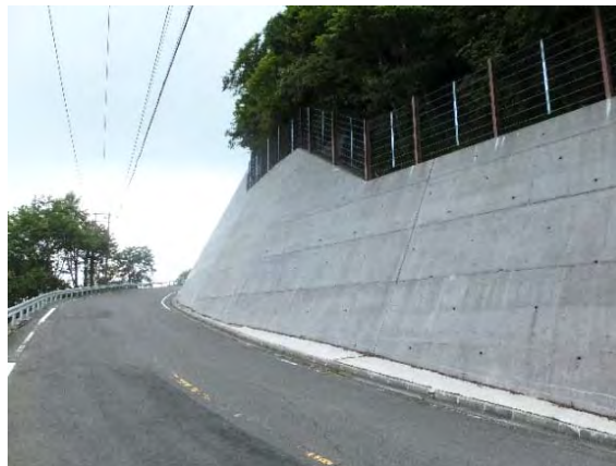
PHOTO 10.2-10 WORKING EXAMPLE OF CONCRETE PITCHING
