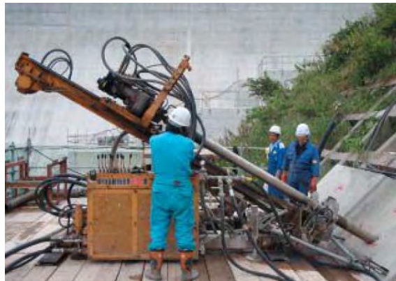
PHOTO 10.2-16 CONSTRUCTION STATUS OF GROUND ANCHOR
