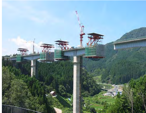
FIGURE 15.5.1-6 BALANCED CANTILEVER CONSTRUCTION METHOD
