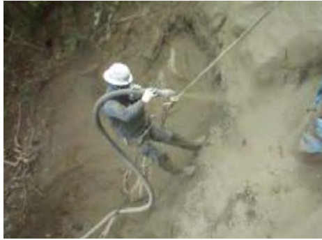
PHOTO 10.2-8 WORKING EXAMPLE OF MORTAR/CONCRETE SPRAYING (SHOTCRETE)
