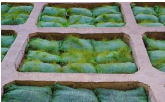
PHOTO 10.2-5 WORKING EXAMPLE OF VEGETATION SANDBAG
