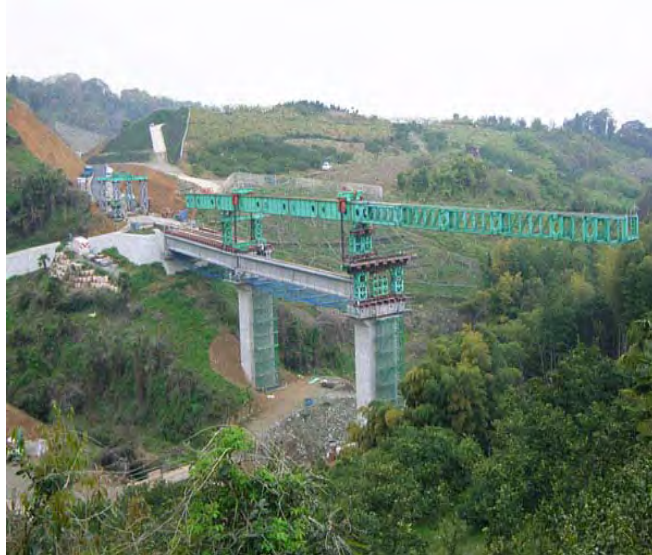
FIGURE 15.5.1-3 DRAW OUT METHOD WITH ERECTION GIRDER
