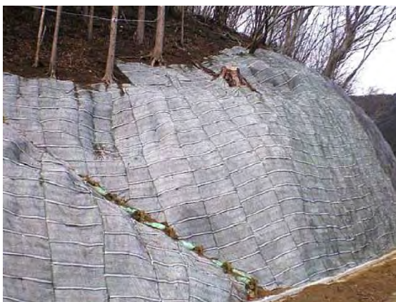
PHOTO 10.2-4 WORKING EXAMPLE OF VEGETATION MAT
