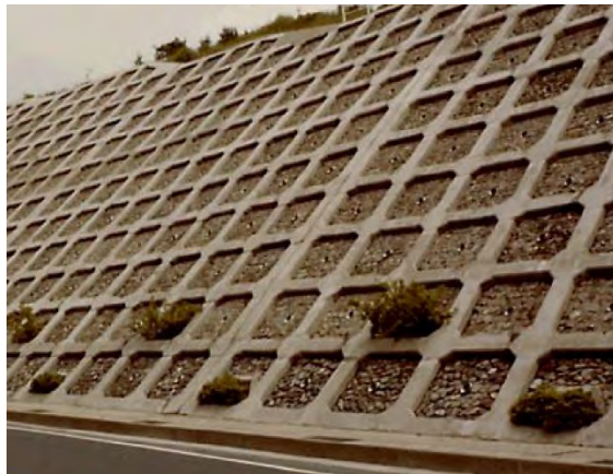
PHOTO 10.2-11 WORKING EXAMPLE OF GRATING CRIB WORKS USING PRECAST BLOCKS
