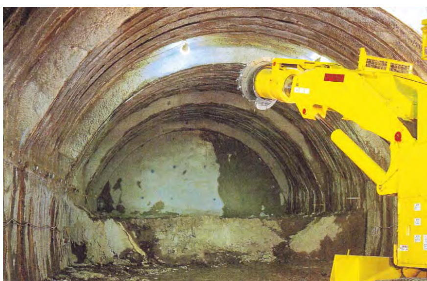
PHOTO 10.4-3 EXCAVATION BY ROOD HEADER
