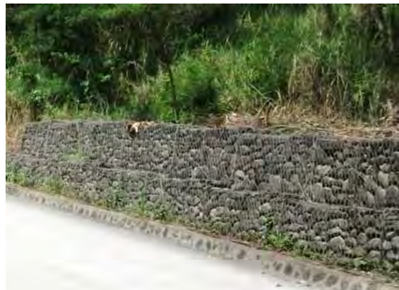
PHOTO 10.2-14 WORKING EXAMPLE OF MAT GABION
