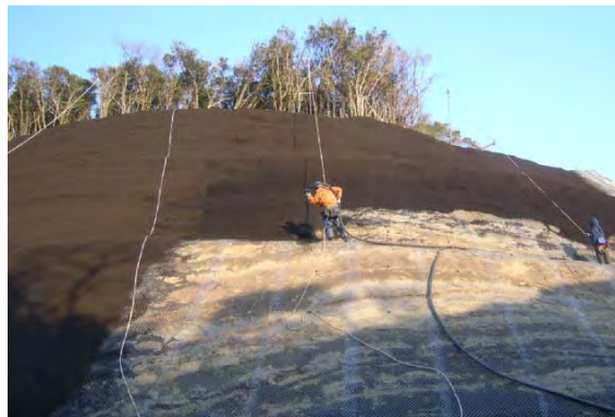
PHOTO 10.2-3 WORKING EXZMPLE OF VEGETATION BASE MATERIAL SPRAYING
