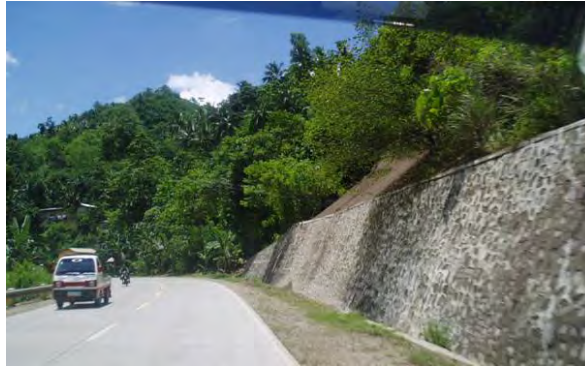
PHOTO 10.2-13 WORKING EXAMPLE OF STONE/RUBBLE-CONCRETE MASONRY
