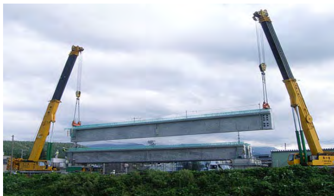
FIGURE 15.5.1-5 ERECTION BY TRACK CRANE
