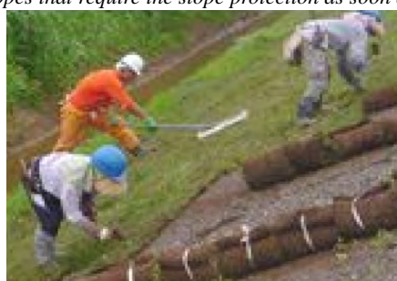
PHOTO 10.2-6 WORKING EXAMPLE OF SODDING
