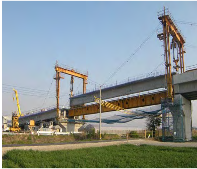
FIGURE 15.5.1-3 DRAW OUT METHOD WITH ERECTION GIRDER
