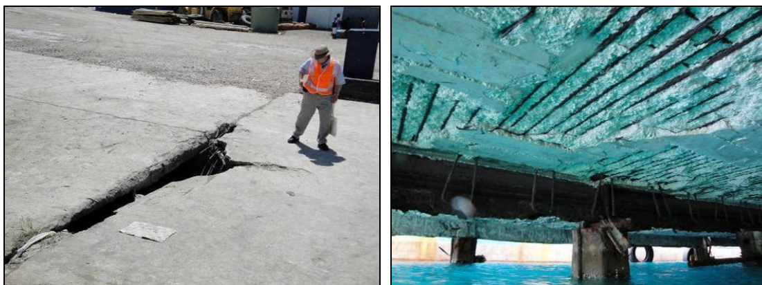
Figure 8: Serious physical deterioration of the existing Star Wharf - Dec 2009 (Source: Raaymakers)
