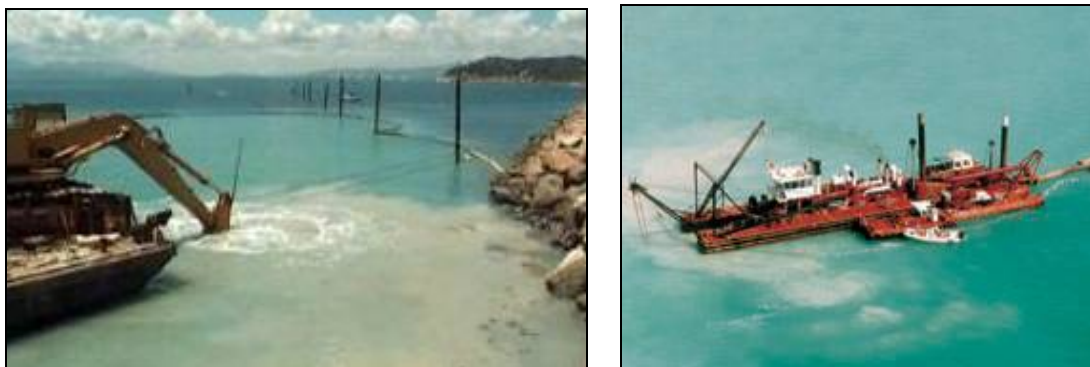
Figure 57: Turbidity from dredging in reef areas. Sediment plumes can impact on adjacent corals and other resources. In the left image a silt curtain can be seen at top right, held in place with stakes. This might be the best method for fixing the silt curtain at the Star Wharf reclaim area (Source: left GBRMPA , right gldd.com)
