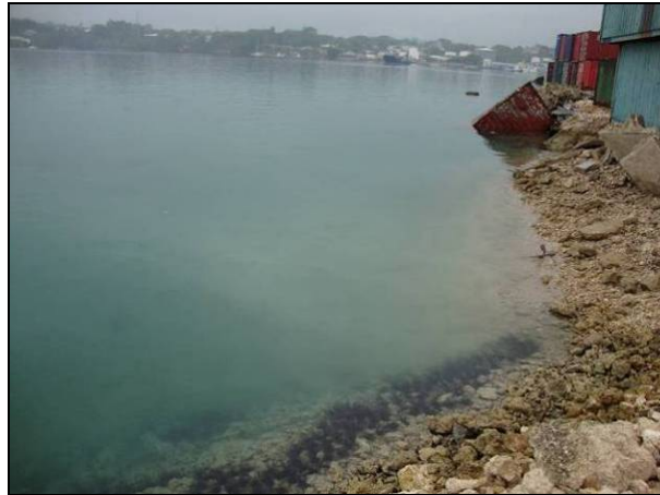
Figure 37: Seepage of fine silts from the porous seaward face of ad-hoc reclamation works at Star Wharf (Feb 2010). Such silts can be detrimental to benthic marine life. The new development will improve this through proper rock armouring of all reclaim faces (Source: Raaymakers)
