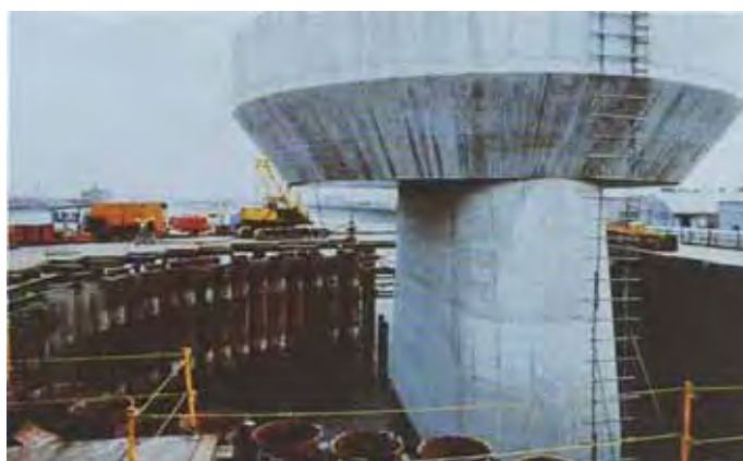
Picture 7.1 Example of Steel Pipe Sheet Pile Foundation
