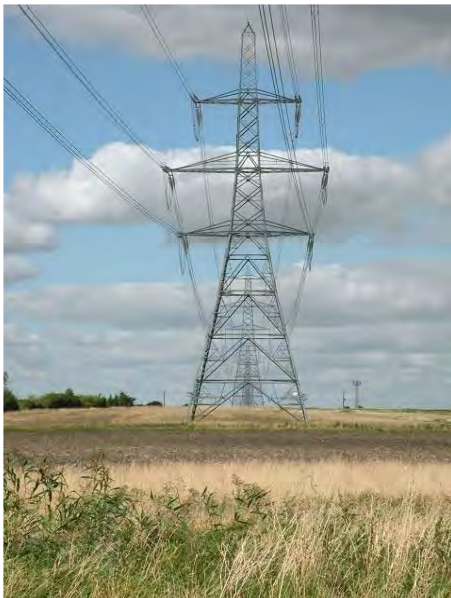
Photo 11: Example of a 400 kV Transmission Line
